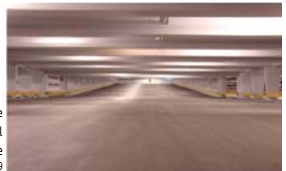
atl one dng hall garage digital photographs 2009
